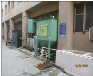
External photo(s) of the production unit(s) EFFLUENT TREATMENT PLANT.JPG
